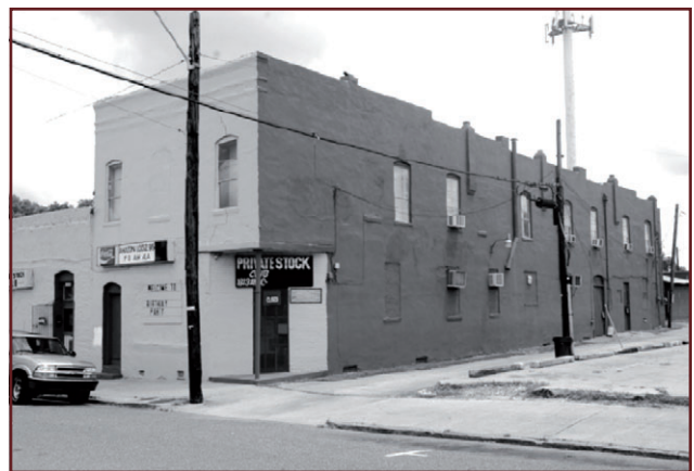
Knights of Pythias Hall, 1913 Avenue C. Little remains of the once-thriving African-American business district that extended along Avenues C and D. This building, built circa 1900, housed the "colored" K of P Hall in the early 20th century.
