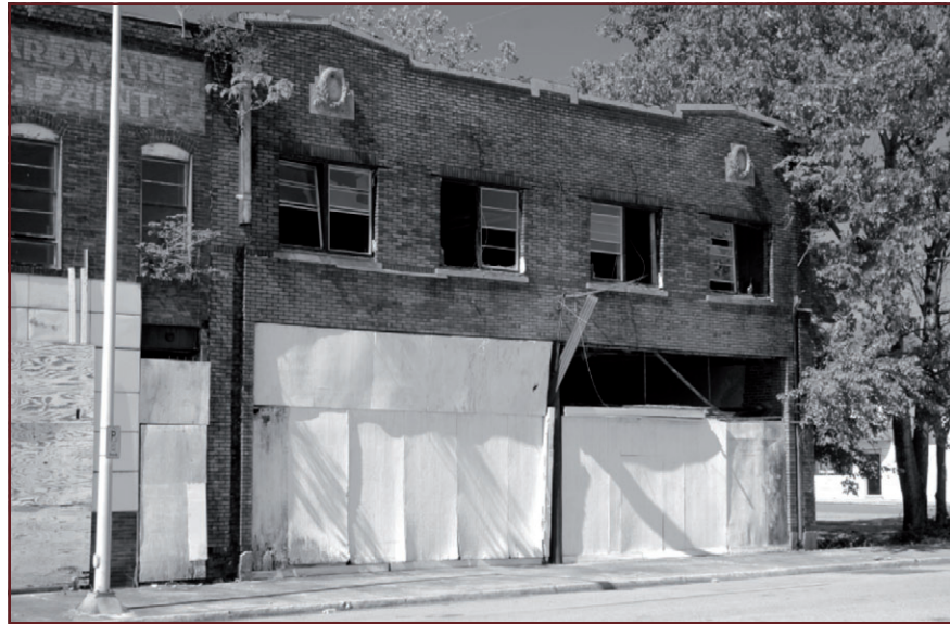
Neglected Commercial Building, 305 19th Street - Many of Ensley's buildings are in an advancing state of deterioration.
