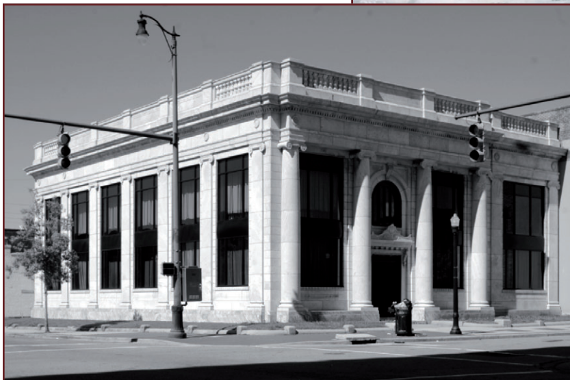
Left Bank of Ensley, 1919, established in 1899 by Erskine Ramsay and George B. McCormack Schneider Historic Preservation, LLC
