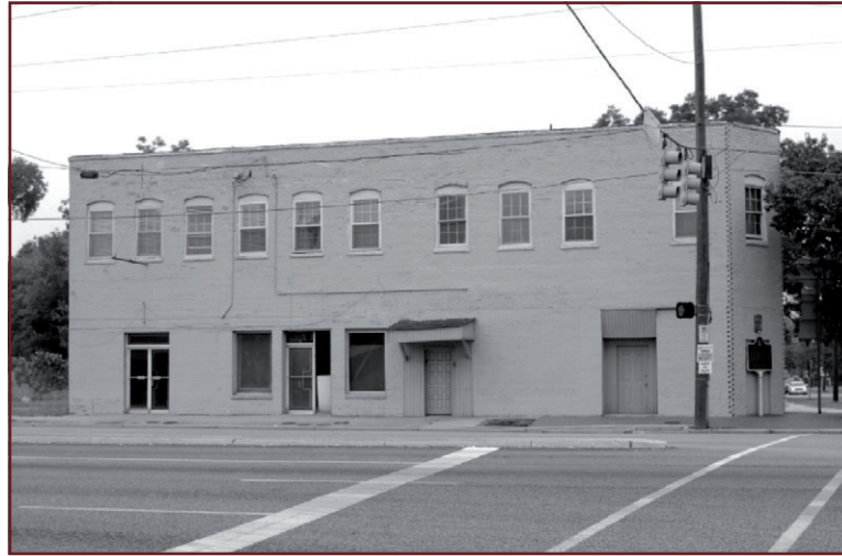
Belcher-Nixon Building in 2008 Schneider Historic Preservation, LLC
