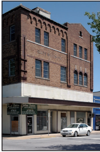
Knapp Building at 600-602 19th St. (survey #039, circa 1910)
