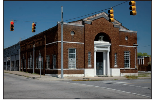
Bank of Alabama (Survey #095)
