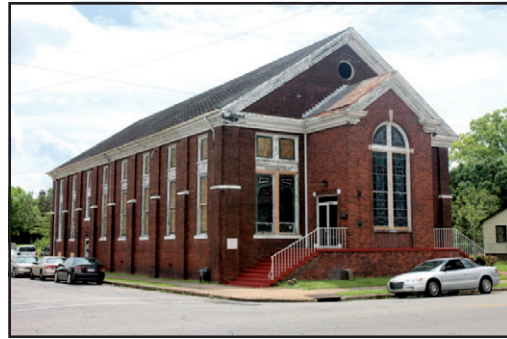
Ensley Christian Church, 2101 Avenue F (survey #155, 1914).
