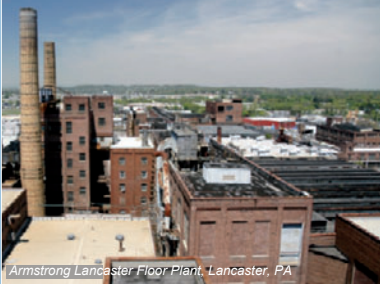
Armstrong Lancaster Floor Plant, Lancaster, PA
