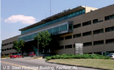
U.S. Steel Pintridge Building, Fairfield, AL
