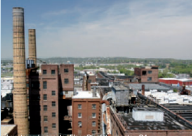
Armstrong Lancaster Floor Plant, Lancaster, PA
