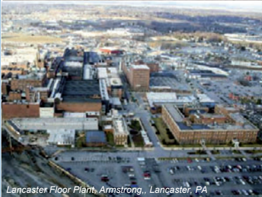
Lancaster Floor Plant, Armstrong, Lancaster, PA
