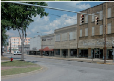
Tuscaloosa Urban Renewal Area, Tuscaloosa, AL
