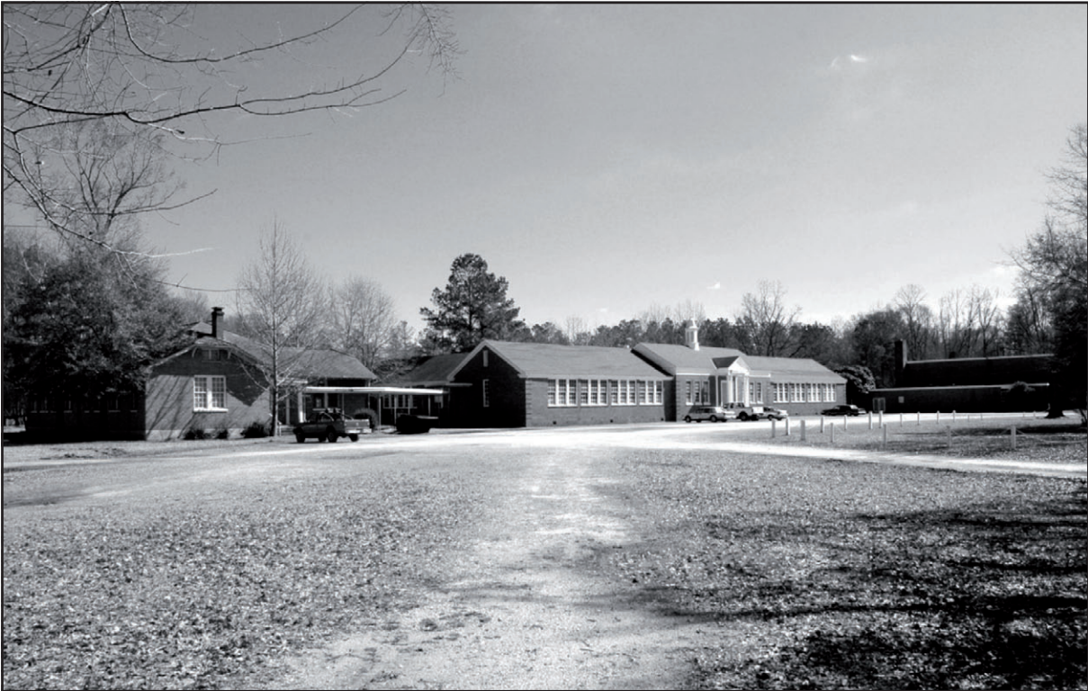
AL_PerryCo_Suttle_0038. Resource #22, camera facing southeast
