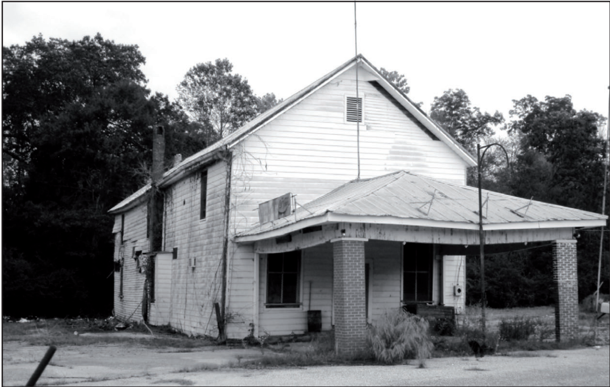
AL_PerryCo_Suttle_0011. Resource #2, prior to demolition, camera facing southeast, photo by MRS Consultants, LLC
