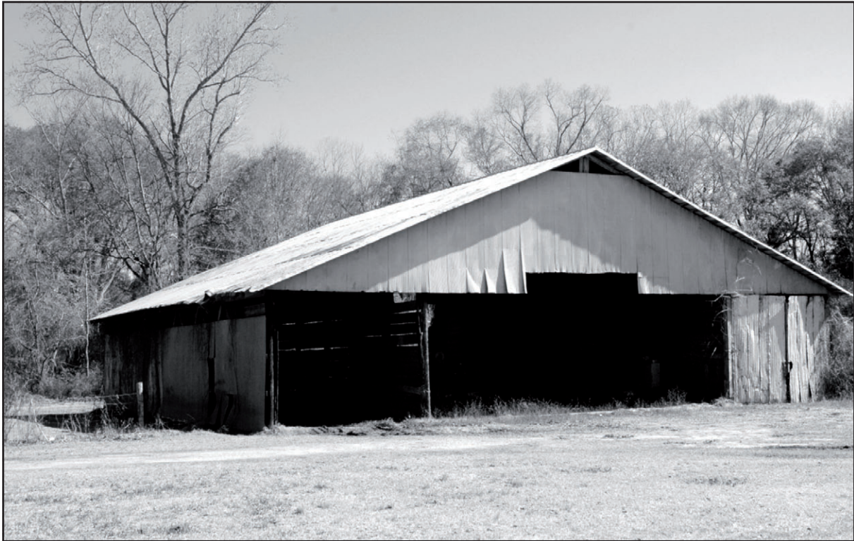
AL_PerryCo_Suttle_0025. Resource #10, camera facing southeast
