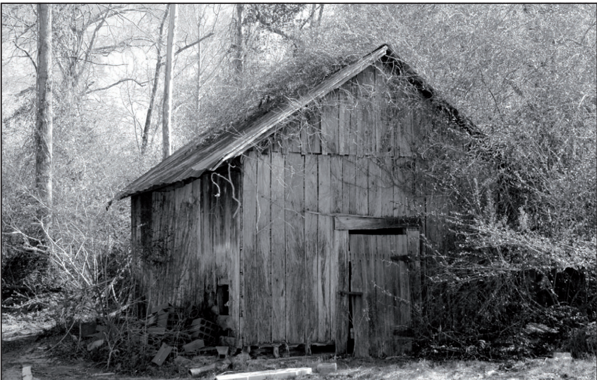
AL_PerryCo_Suttle_0014. Resource #2, detail of shed, camera facing southeast
