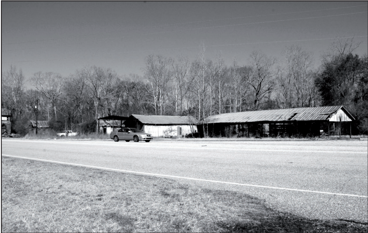
AL_PerryCo_Suttle_0005. Streetscape along Alabama Route 14, Resource #1, camera facing northeast
