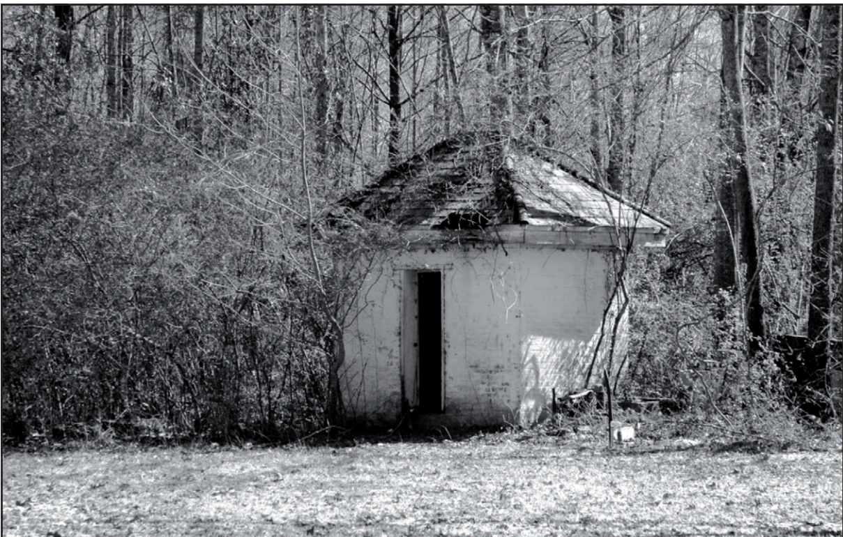
AL_PerryCo_Suttle_0028. Resource #12, well house, camera facing southeast
