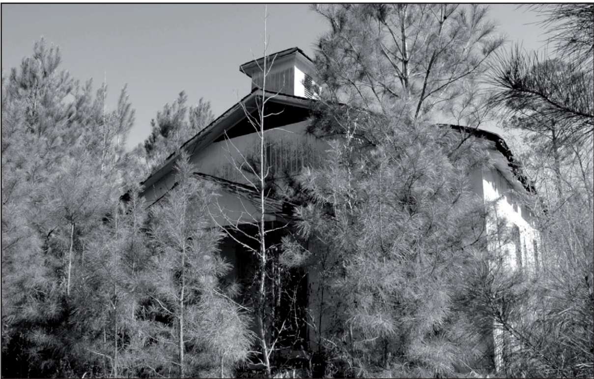
AL_PerryCo_Suttle_0035. Resource #19, camera facing northeast
