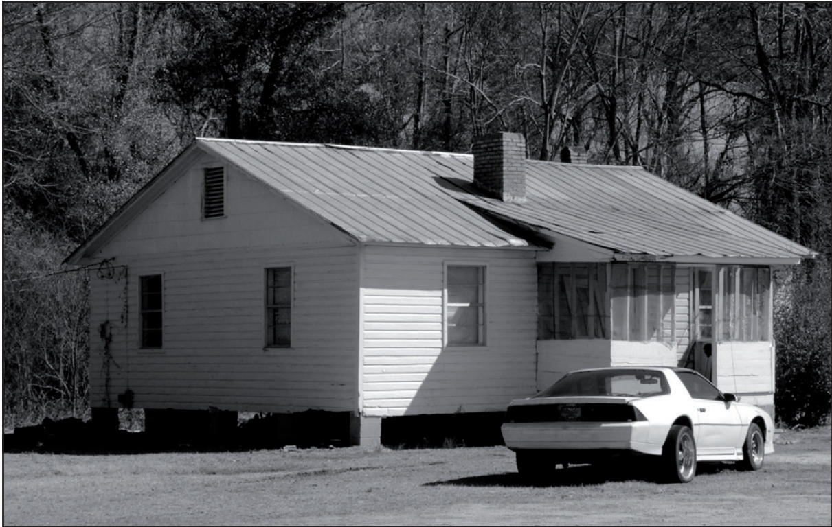
AL_PerryCo_Suttle_0030. Resource #14, camera facing southeast
