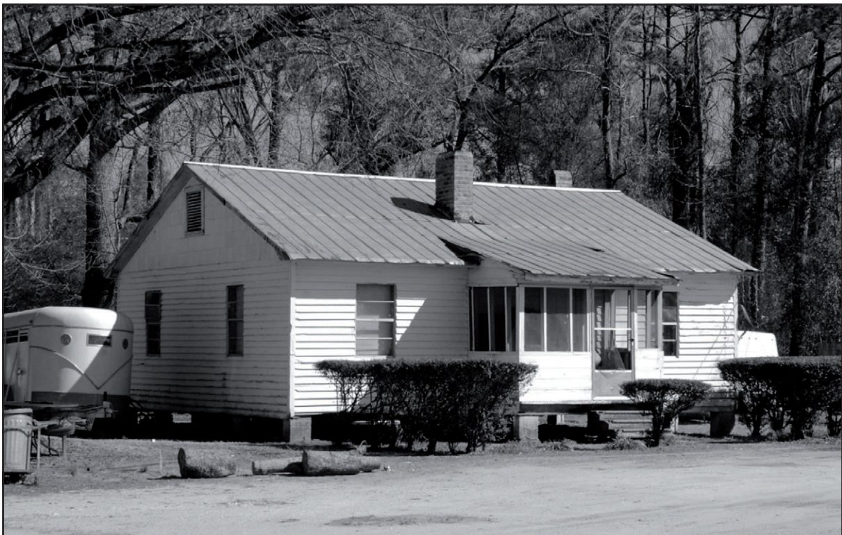
AL_PerryCo_Suttle_0031. Resource #15, camera facing southeast
