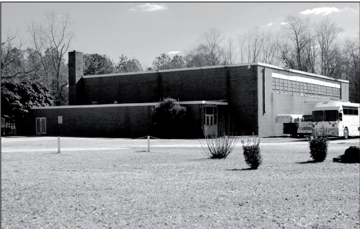
AL_PerryCo_Suttle_0044. Resource #22, gymnasium, camera facing southeast
