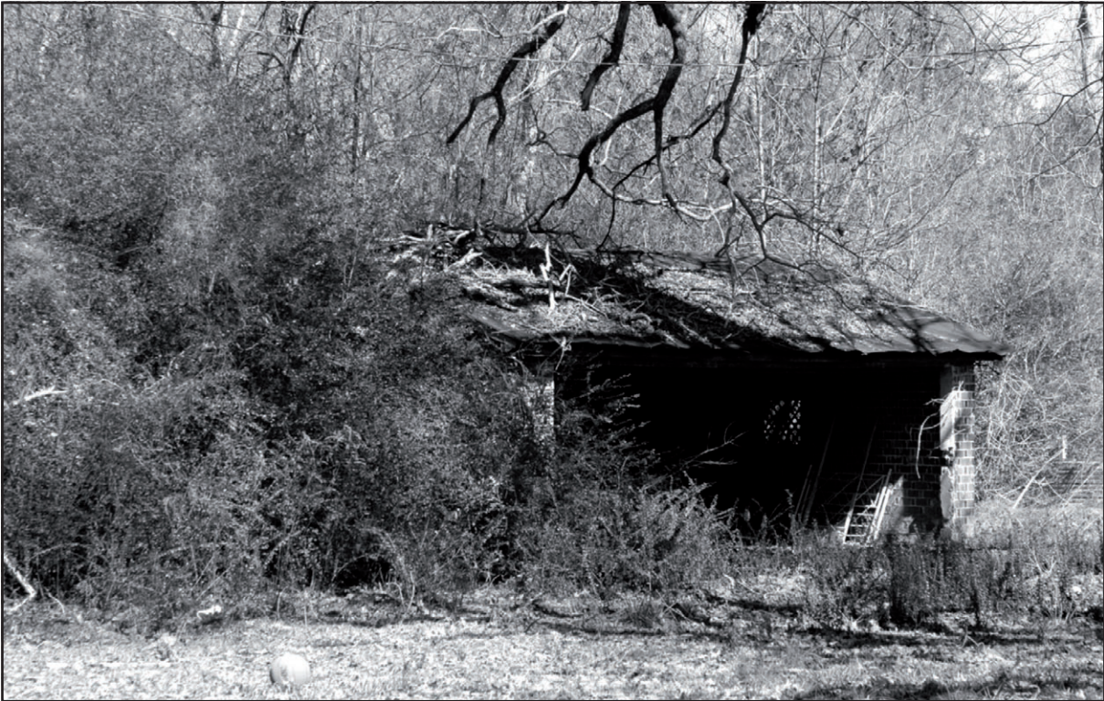
AL_PerryCo_Suttle_0027. Resource #12, garage, camera facing northeast
