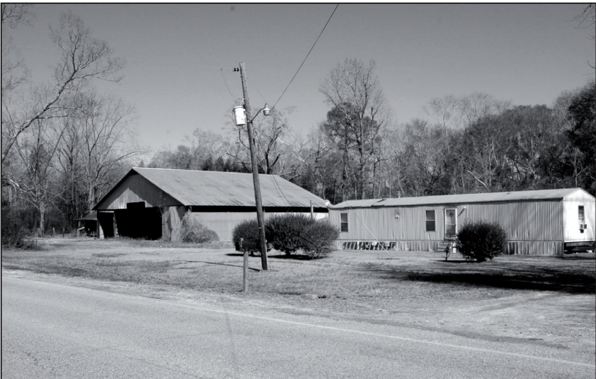
AL_PerryCo_Suttle_0020. Streetscape along Alabama Route 14, Resource #10, camera facing northeast
